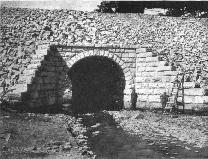
Stone Arch Culvert 6.00 Meter, at Kilometer 77 State of Chihuahua, Mexico.
